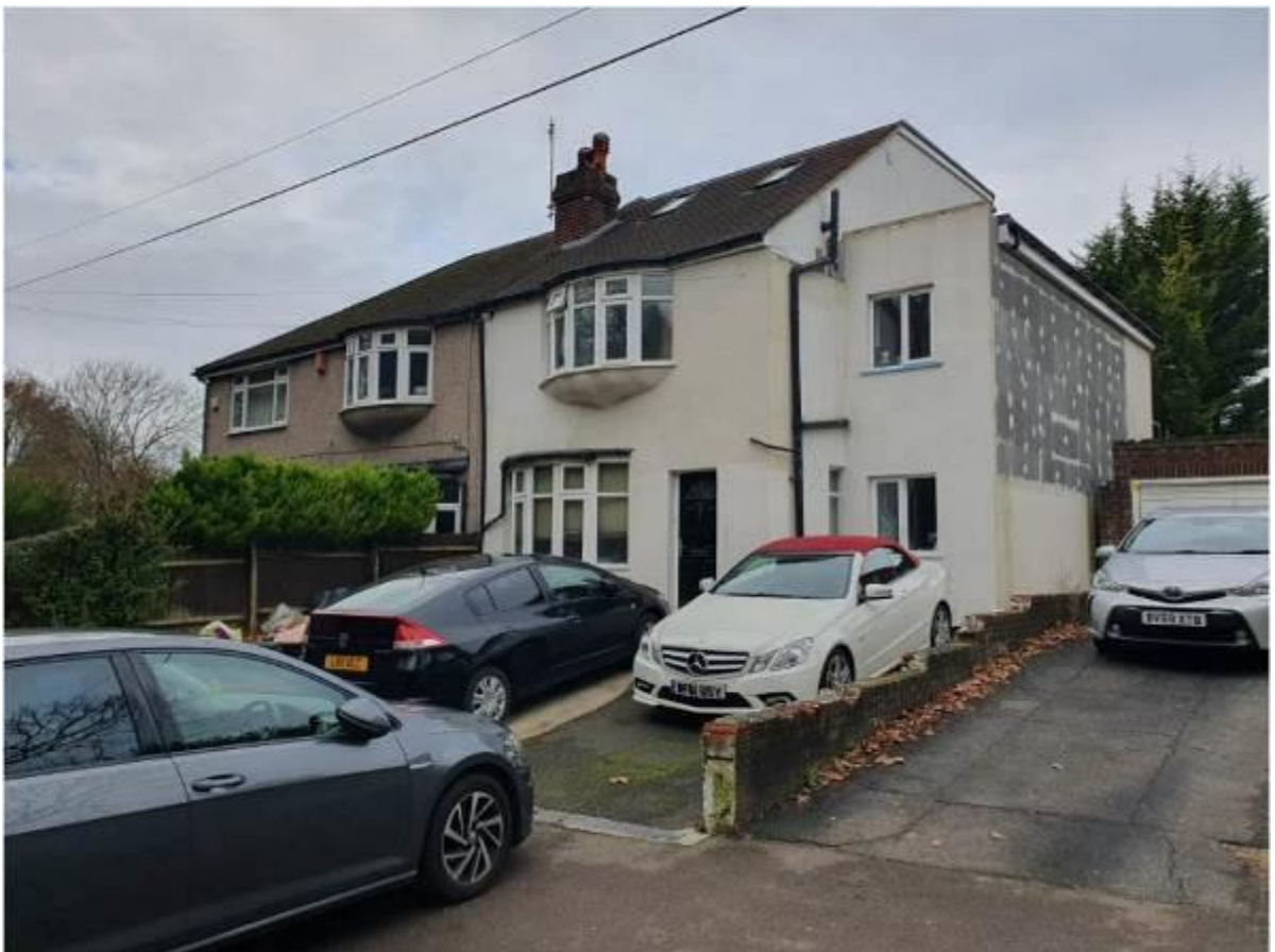
Figure 6: Photographs of the site from the front:
